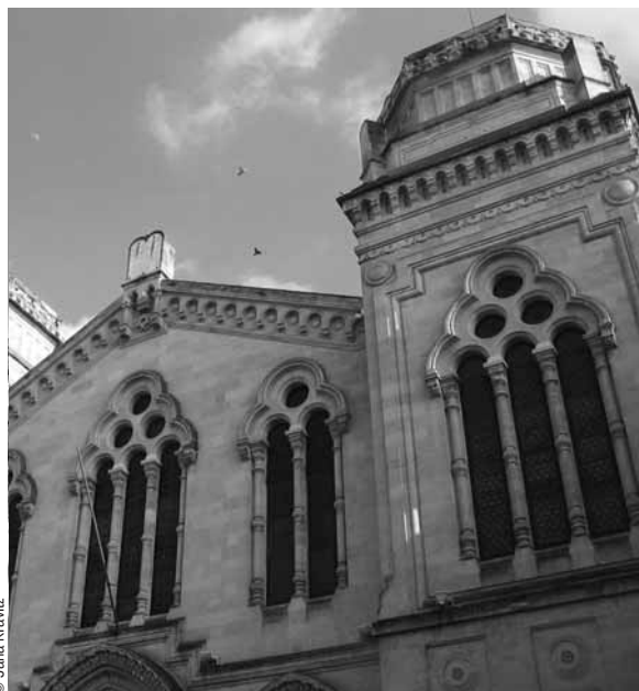
The central façade of the Bordeaux Synagogue, the largest in France (Aquitaine)
